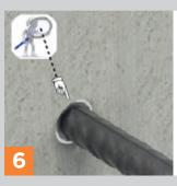
When installation is complete check no threaded portion of the rebar is visible outside the coupler.
