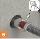
Check the distance "I" between the coupler and lock nut (still engaged at the bottom of the long thread) it has to fall between the limits indicated in table 3 below.
