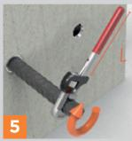
Tighten the joint using a wrench on the continuation bar.
