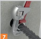
Set the rebar in the correct position and use a wrench to tighten the lock nut.
