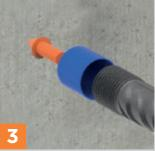
Remove the plastic protection from the 2nd phase rebar.
